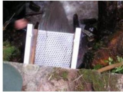
Flat screen in road culvert
